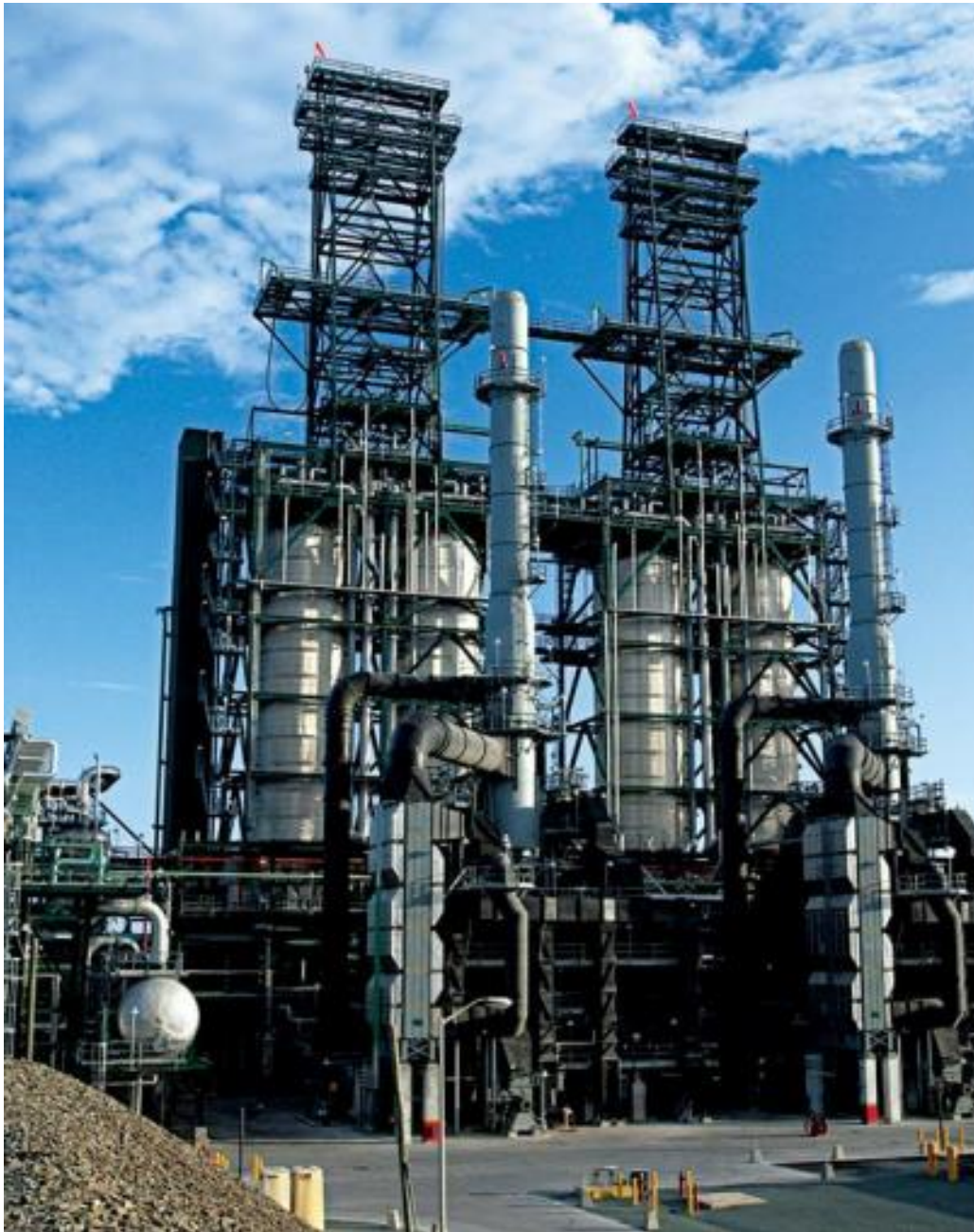
A 4-drum delayed coking unit in a petroleum refinery
