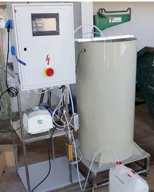
Figure 2. Membrane bioreactor pilot plant.
