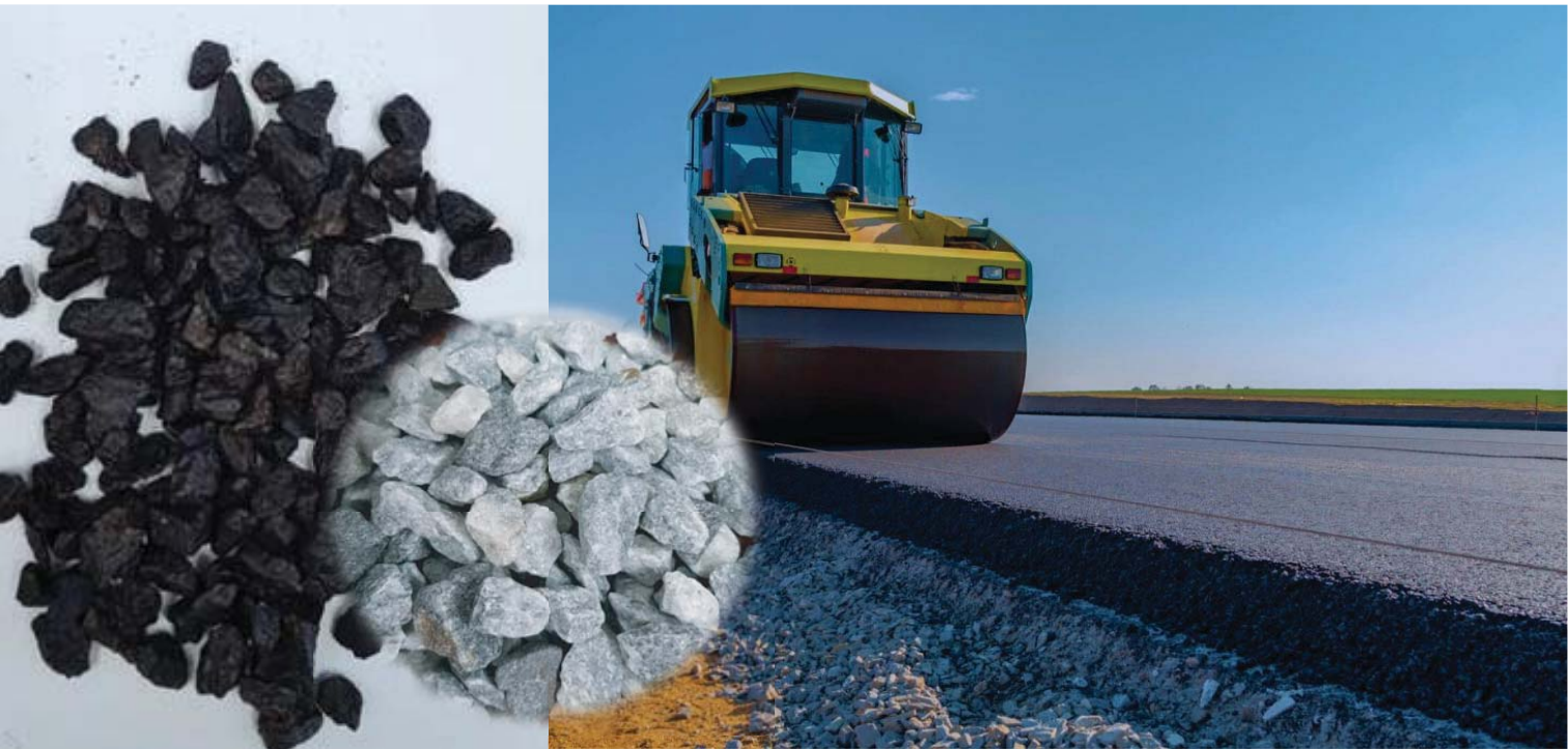
Figure 1. Use of bitumen primer in road construction.
